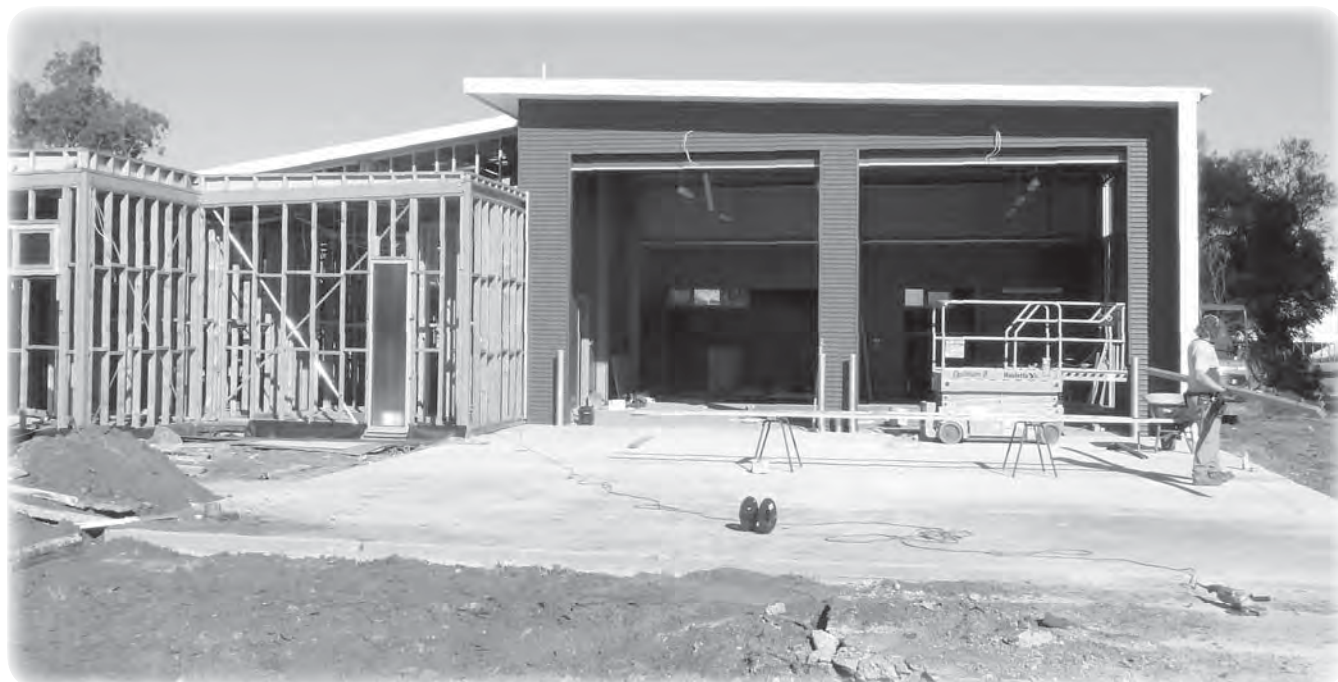
Construction underway at the Berrivillock Multipurpose Community Centre.
